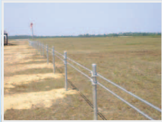
FIXED BOLLARDS REQUIRED FOR ALL CORNER INSTALLATIONS
