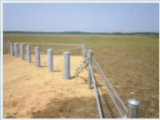
CONTINUOUS TURNBUCKLE TENSIONING ADJUSTMENTS REQUIRED UTILIZING 3/4" CABLES
