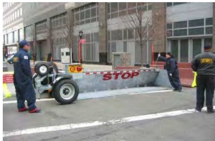
Figure 6-4 Maximum Security Vehicle Arrest Barrier (Example 4)
